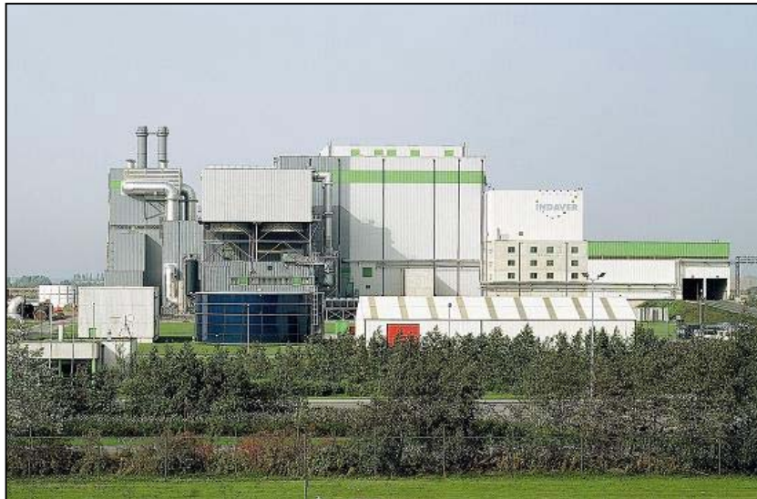
Figure 1.0 : Indaver NV Waste to Energy Facility in Belgium
