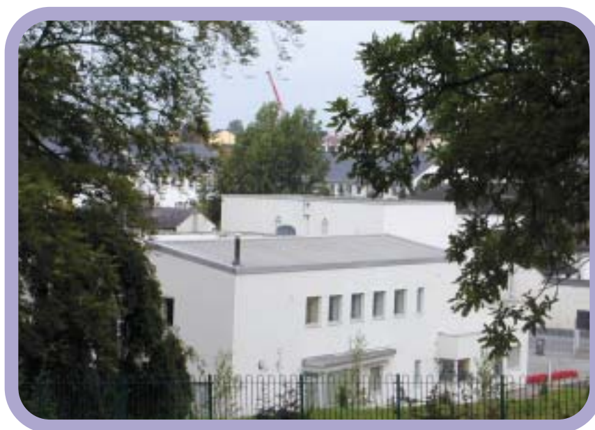
Figure 16 – Navan Education Centre – VSAT Satellite
