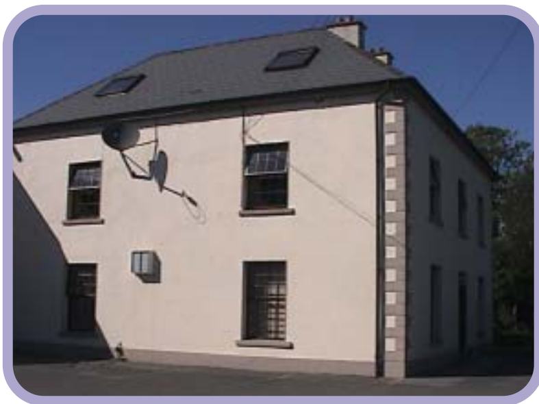
Figure 15 – The Kilcormac Community Centre – VSAT satellite
